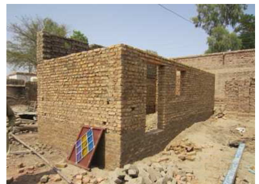
Shelters in various stages of progress in Beero Khan ghadi
